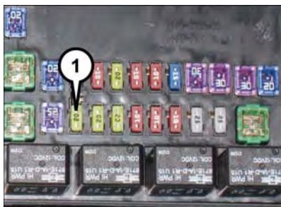
Rear Quarter Power Outlet Fuse
