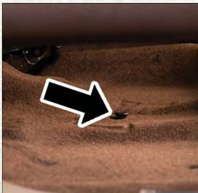
Floor Fastener Location
